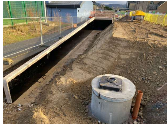
Retaining wall completed
