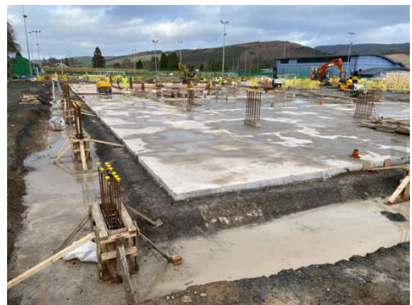
Blinding concrete to floor slab
